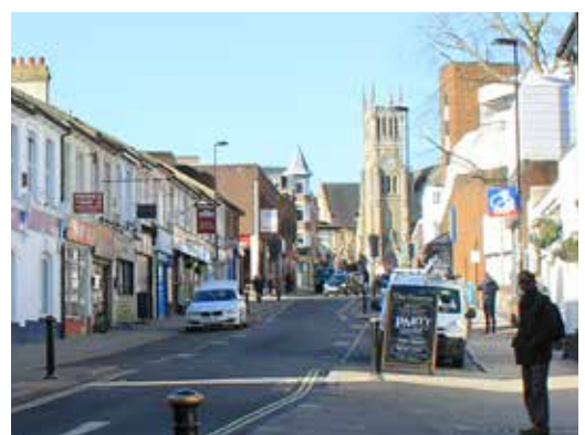
View of Wesley Chambers east along Victoria Road
